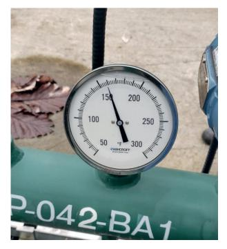
Fig. 8. Ashcroft Bimetallic Thermometer.
