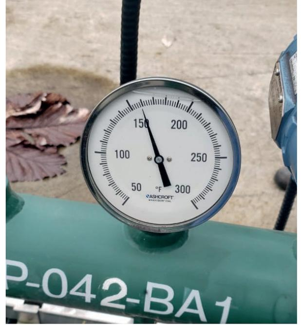
Fig. 8. Ashcroft Bimetallic Thermometer.
