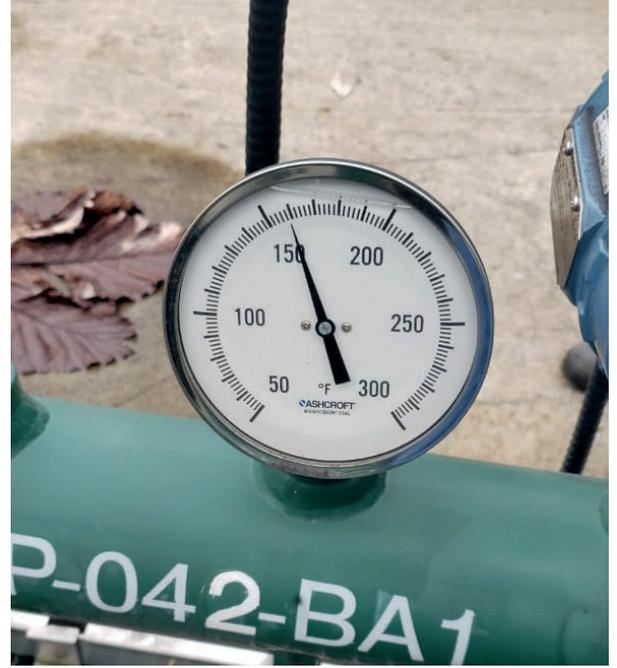
Fig. 8. Ashcroft Bimetallic Thermometer.
